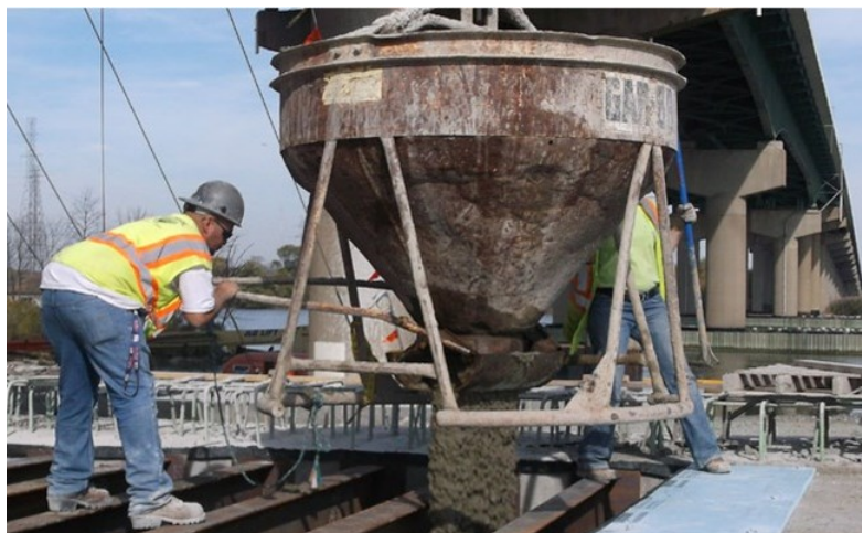
Repair work for the I-495 Bridge in Delaware
