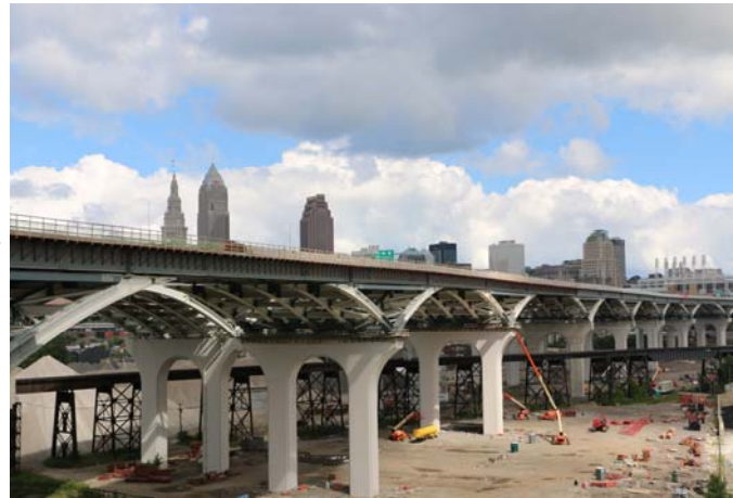
A view of the eastbound bridge when it was near completion in September 2016.
