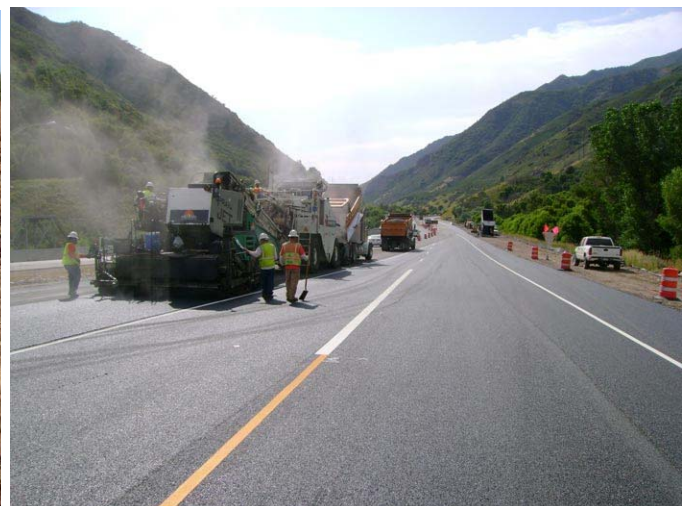
Repaving project in Arizona
