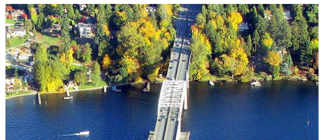
Figure 1: State Route 520 Bridge in Seattle, Washington (Source: Ramanathan)
